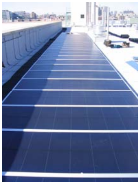
30kW rooftop photovoltaic array was the first solar energy installation in the Bronx
