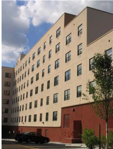
Exterior view of Taino Plaza, Bronx, NY
